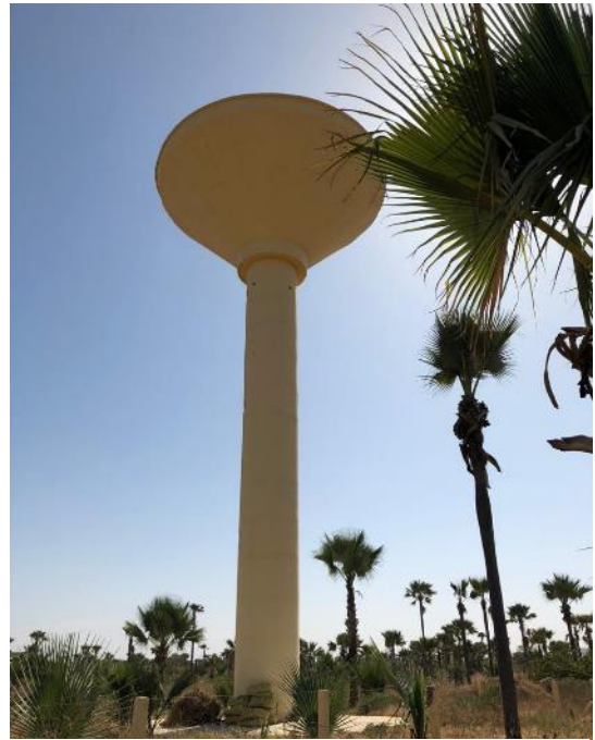
Figure 33 - PUDC Water tower
